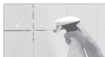
6. Apply a small amount of cleaning agent to the joints. Note the application times recommended by the manufacturer.
